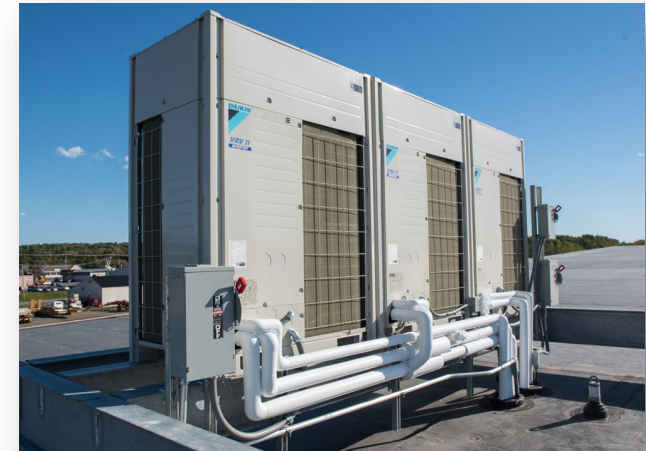
Presque Isle Community Building
